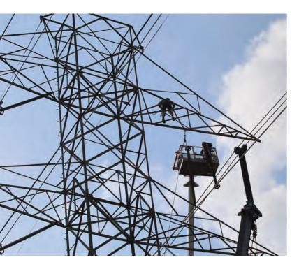
bonded to the conductor, putting them at the same potential as the energized conductor allowing them to physically touch the energized conductor and equipment. To support conductors while unclipping or clipping, the LineMaster Single Point Lifter robotic arm was used. This tool provided safe, secure and controlled support of the energized conductors.
